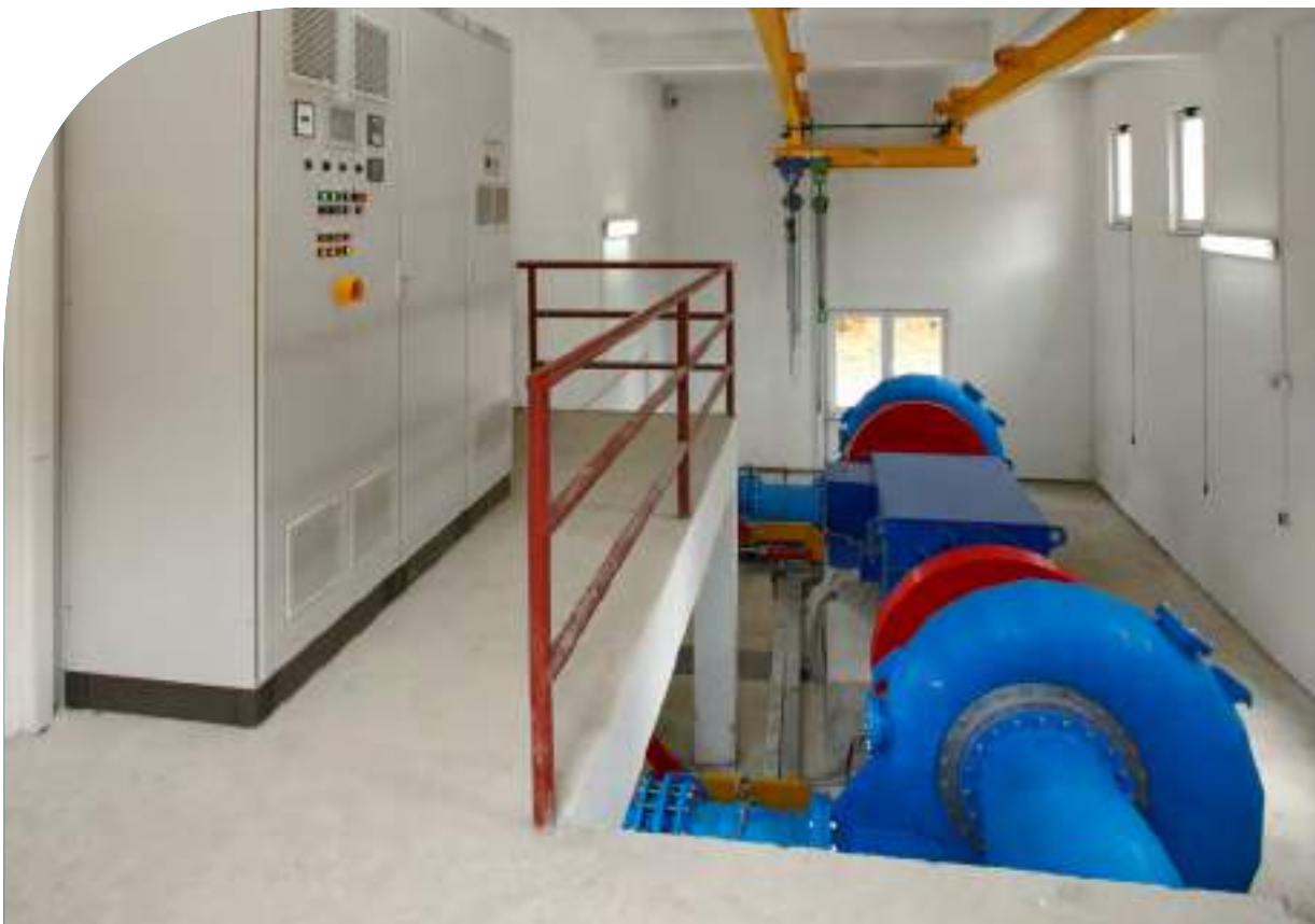
SHPP in Bosnia and Herzegovina
