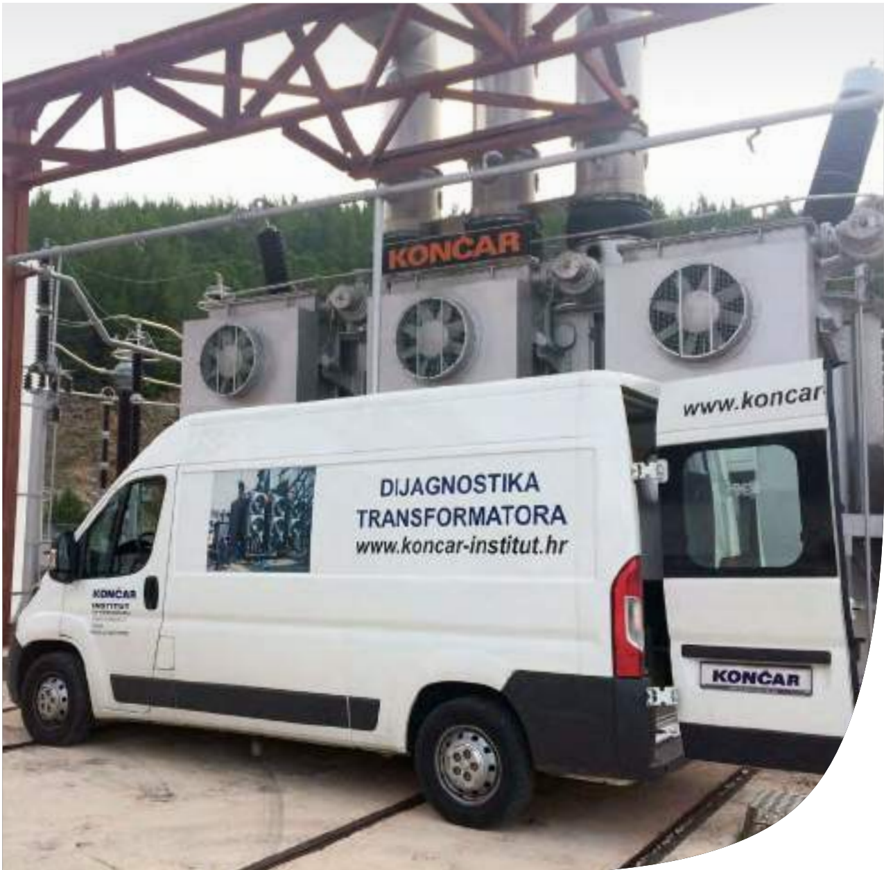
Transformer and reactor diagnostics, servicing and repairs
