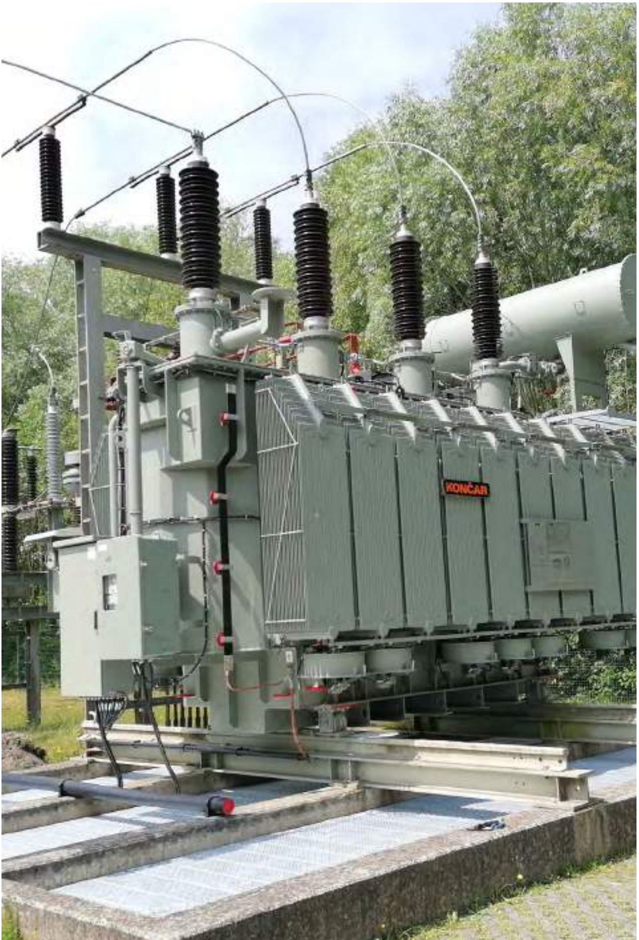
Three-phase oil immersed transformer, rated power 40 MVA
